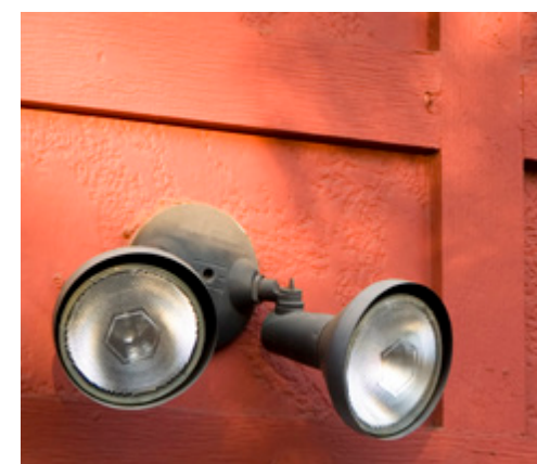
Replace old outdoor fixtures with ones that are motion- or light-activated. And position them high enough so they can't easily be disabled.
